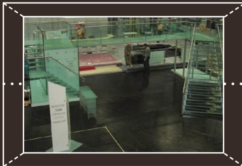
Setting-up the staircase
